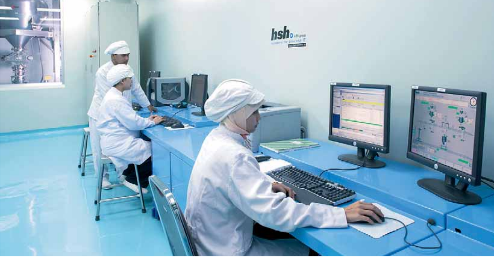
Central control panel with process management and visualisation system
